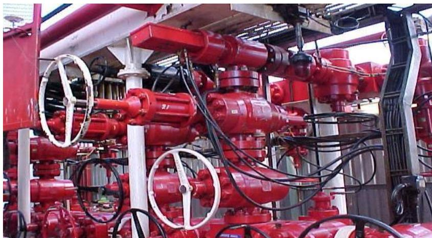
Figura 84: Arranjo do choke manifold
