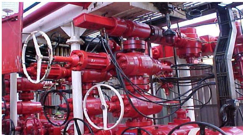
Figura 84: Arranjo do choke manifold
